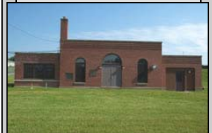
Facility #3 (Ground Water) .864 MGD by Permit
