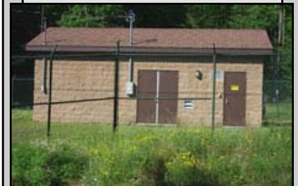
Facility #2 (Ground Water) 1.152 MGD by Permit
